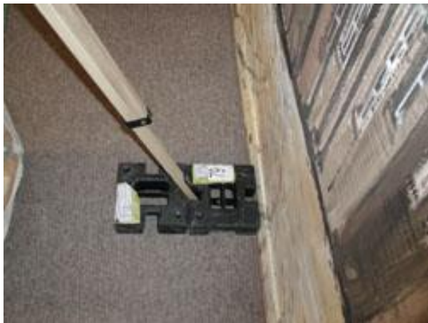
The two weights rest either side of the pole and up against the back wall of the stage
