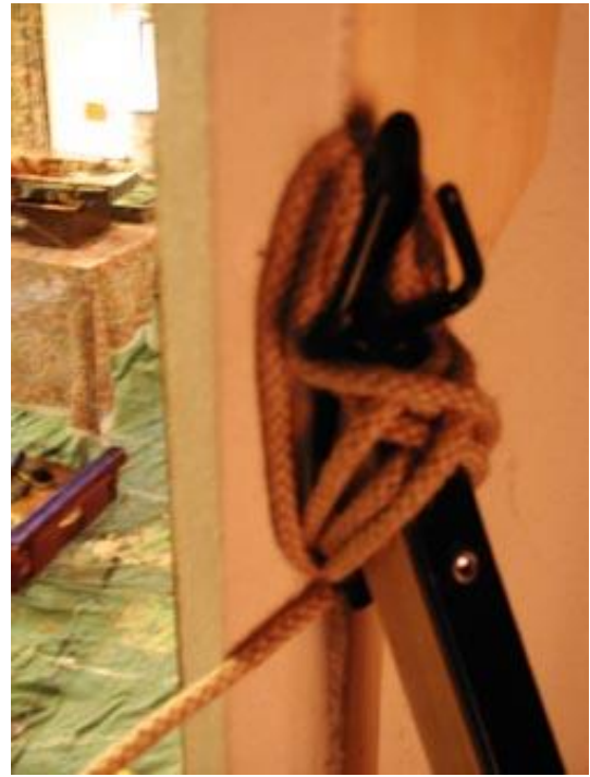
Attaching the pole to the box set for bracing
