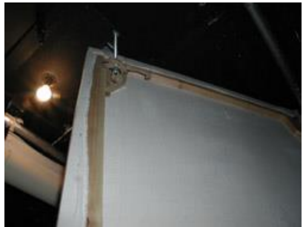
In this example, the arm used for the SL back grey leg was taken off and the metal rod attached to the ceiling was used for extra bracing
