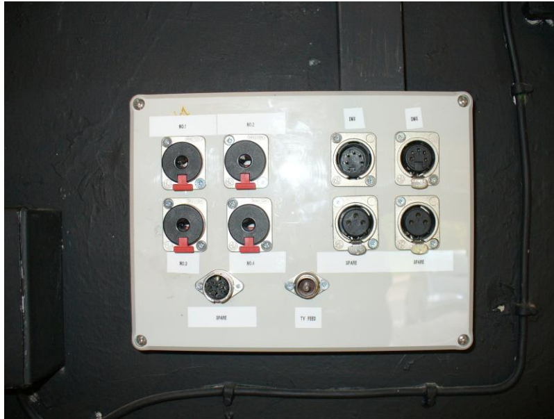
Stage left SM side, patch panel
